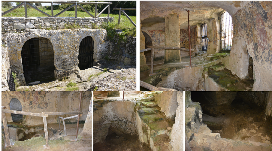
Fig. 1. Sant'Angelo church. Top row: entrance and upper floor. Bottom row: details of the structure.
