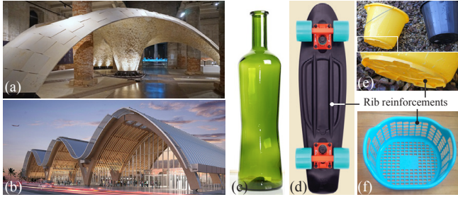
Fig. 2. Examples of shell structures showing variable thickness walls and ribs: (a) The Armadillo Vault, Biennale d'architecture 2016, has thicknesses varying from 5cm to 15cm (Image by Jean-Pierre Dalbéra [2016]); (b) Mactan Cebu International Airport, Philippines (Image by Denzeldoorn [2019]); (c) glass bottle of variable thickness (Image by Dmitry Makeev [2006]); (d) plastic skateboard weights 1.75kg and supports 100kg (Image by MthwGlm [2020]); (e) plastic pails (Image by Davie Bicker [2019]); (f) plastic laundry basket (Image by Dodger67 [2013]).
