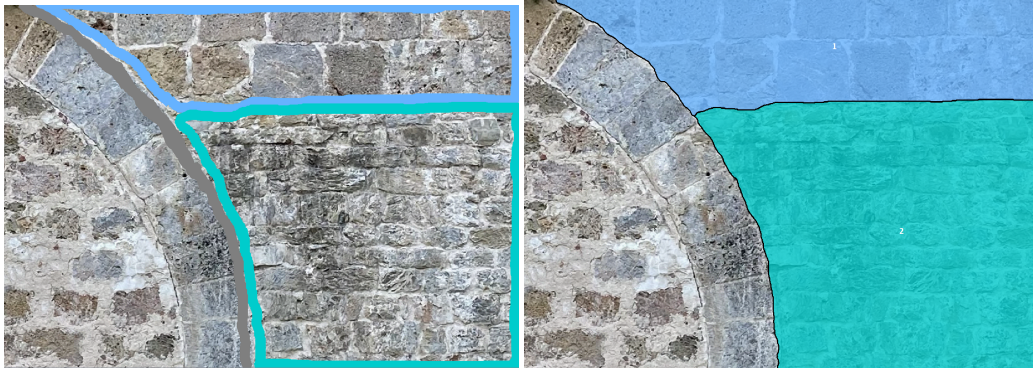
Fig. 5. The Watershed tool in action. The azure and cyan scribbles mark two areas belonging to specific classes, while the grey scribble marks a “background” area to be ignored. The watershed algorithm transforms the scribbles into segmented areas.
