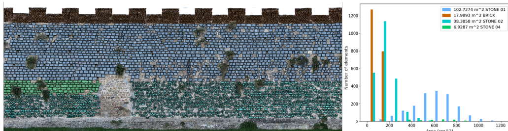
Fig. 13. The bricks segmentation tool automatically traced 6169 bricks in the the ortho Vittorio Veneto A , working on the STONE 01, STONE 02, STONE 04 and BRICK semantic classes, previously detected in Fig. 1. STONE 02 has hardly detectable bricks due to their small size and the white mortar's presence that confounds the outlines. The histogram shows the area of elements identified for each class (in cm^2 ) on the abscissa while the ordinate reports the number of elements.
